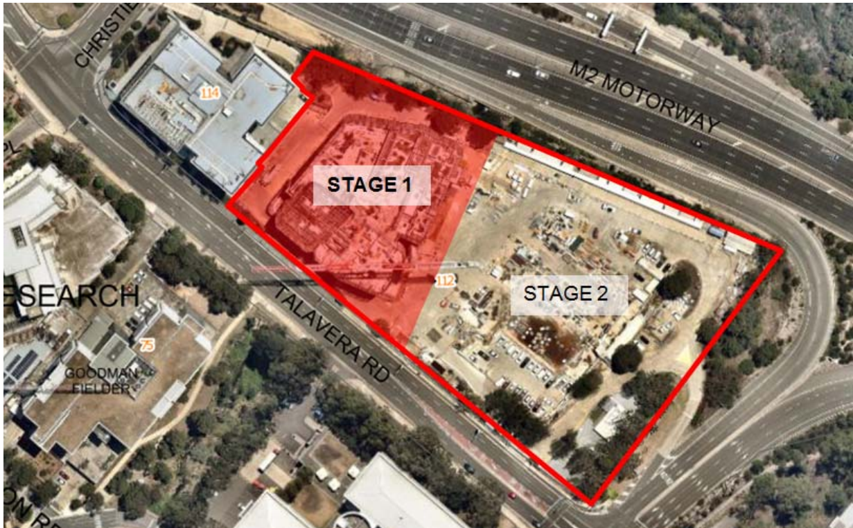
Figure 1: Aerial of the broader site (red outline) and Stage 1 development site (red shading)
