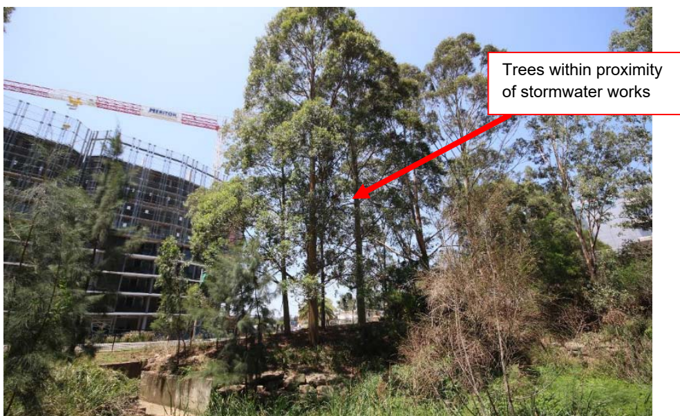
Figure 3: Photograph of trees within University site
